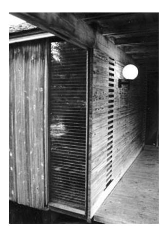
Image 4 - Ventilation strips at wall
